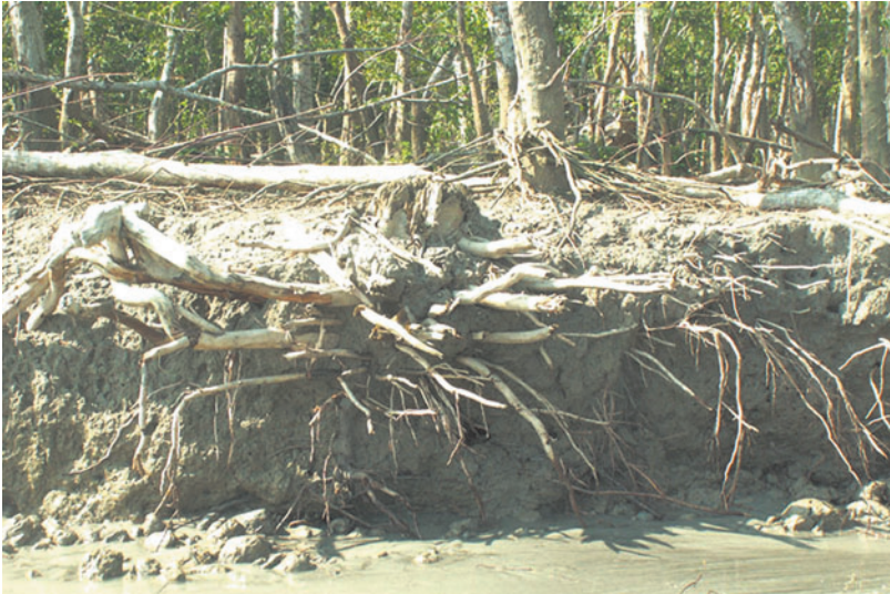
Figure 6. Section of the delta clay and a rooted tree with its horizontal roots spread just below the mud surface (from the western side of the shore segment investigated)
