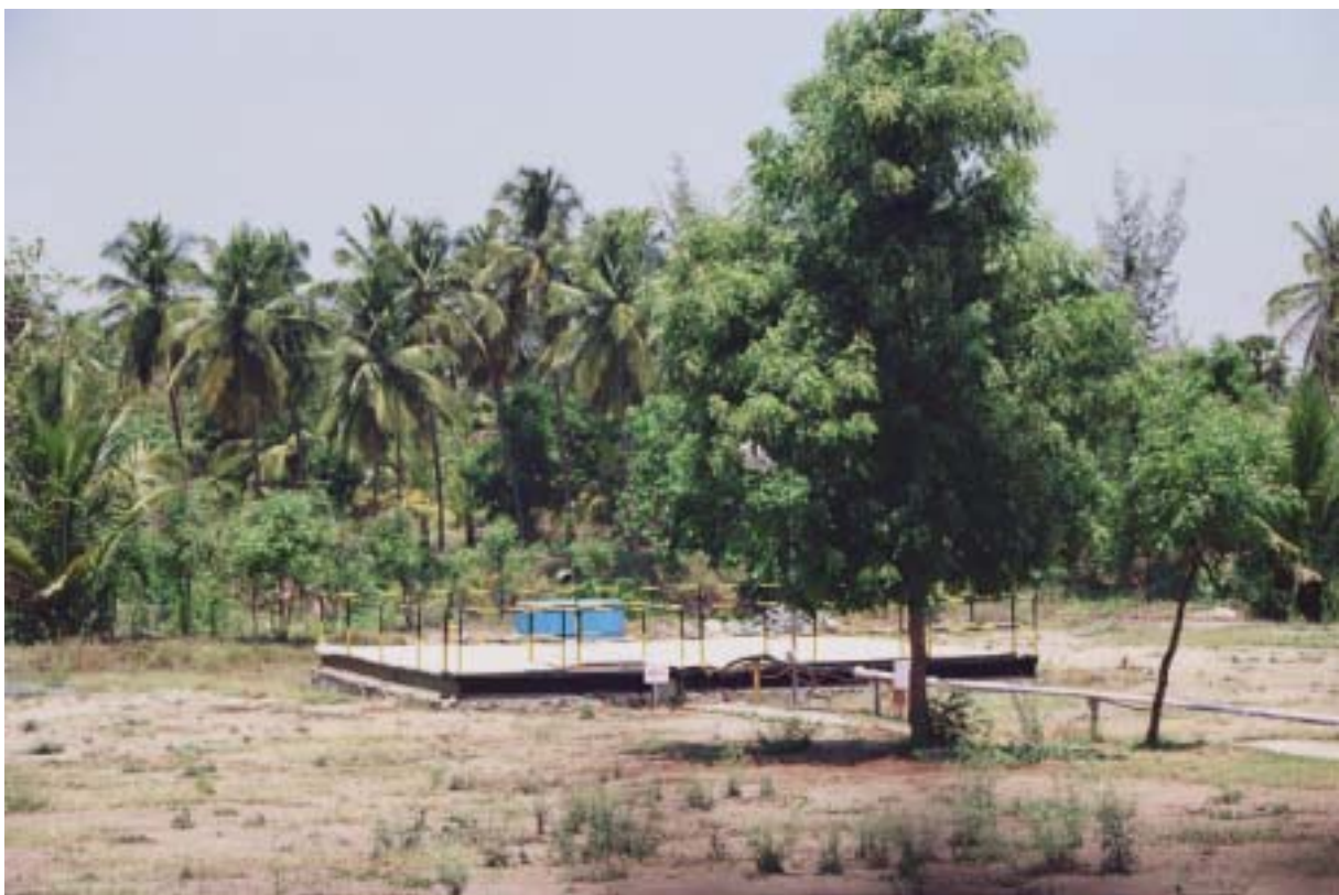
Tank for storing the solid waste inside the Coca-Cola premises (Photo by author).
