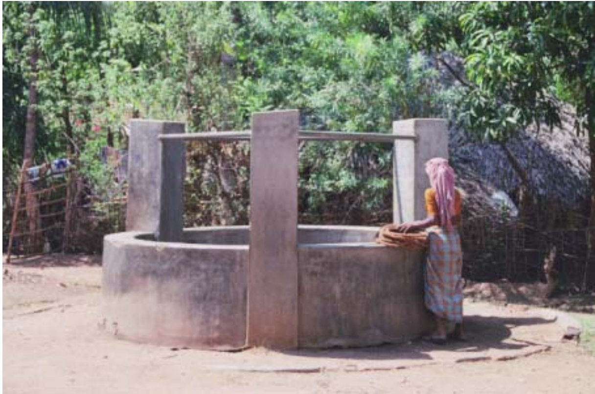
Public well in Plachimada. The horizontal bars are used to make it easier to wind up of the water pot by pulling the rope drawn over the bar. (Photo by author).
